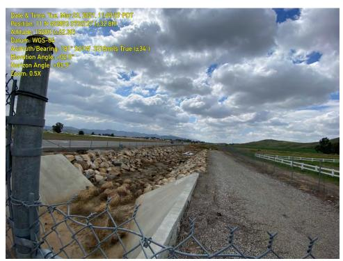
**PHOTOGRAPH 10:** An offsite flood control channel. The southern area consisted of an earthen channel with riprap then transitioned to a concrete channel.
